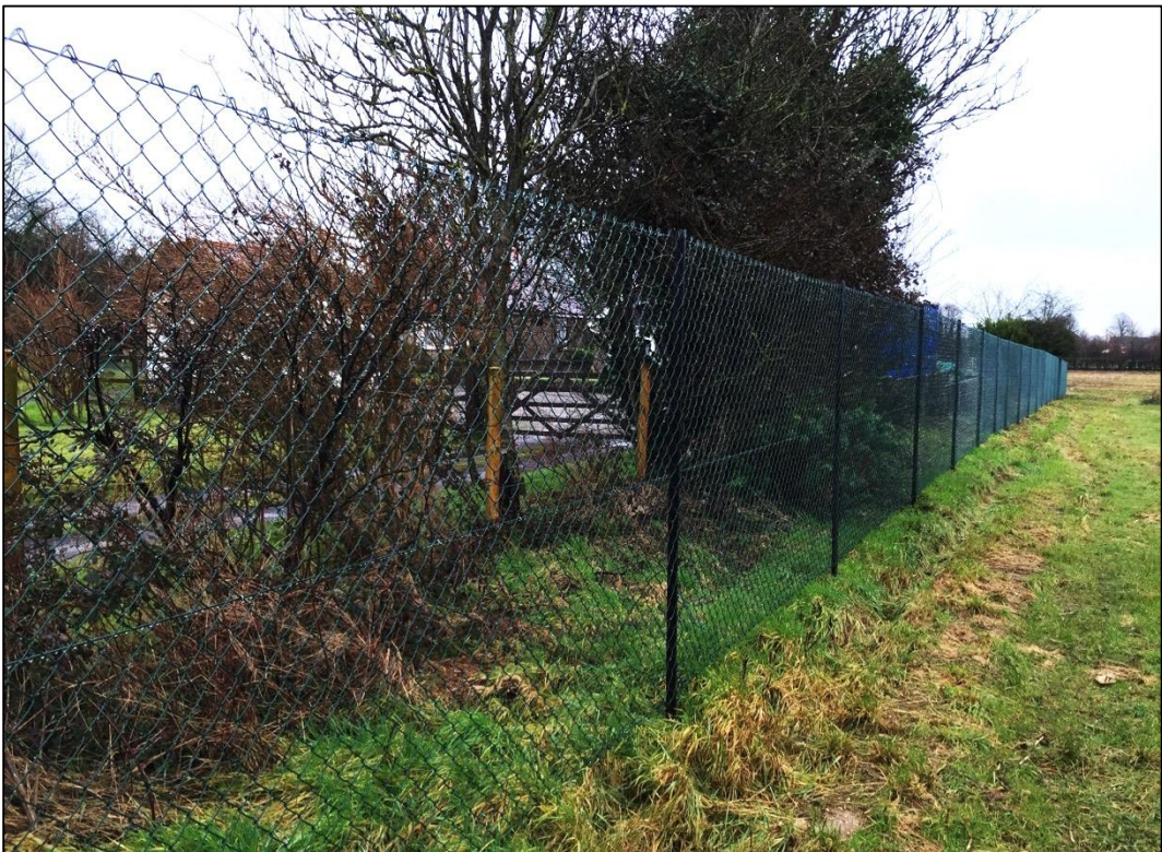
Chain-link on angle-iron uprights
