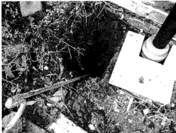
Photograph 2 – Close up of footing in TP1.
