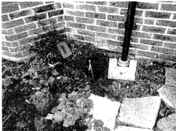
Photograph 1 – View of TP1 position.
