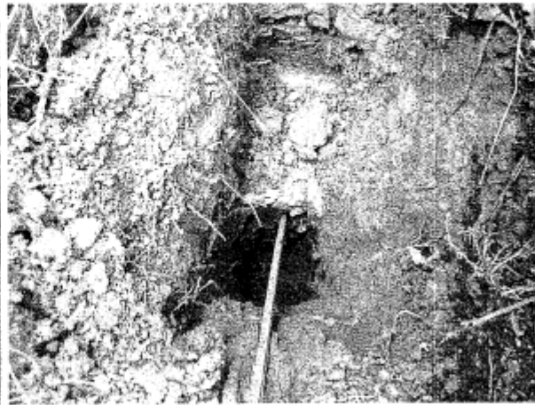
Photograph 6 – Close up of footing in TP3.
