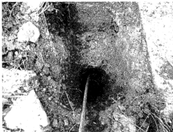
Photograph 4 – Close up of footing in TP/BH2.
