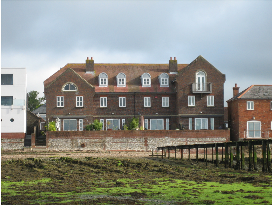
Fig 3 – View of the terrace of 1-4 John King Shipyard from the harbour. The reduced height gable and arched window of No. 1 is clearly visible.
