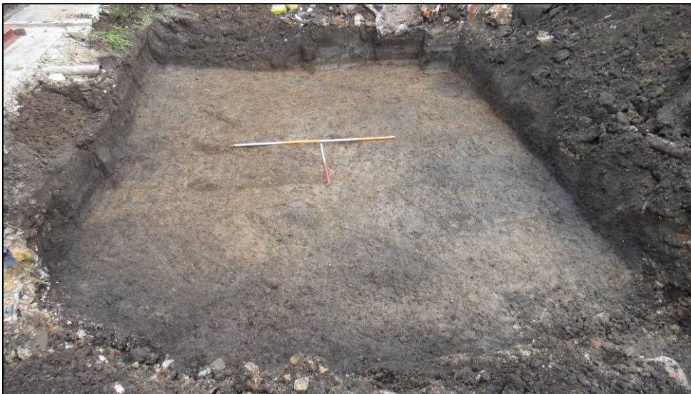
Plate 45. Phase 2a area stripped, looking E; scales 2m & 1m (photo 1/31)
