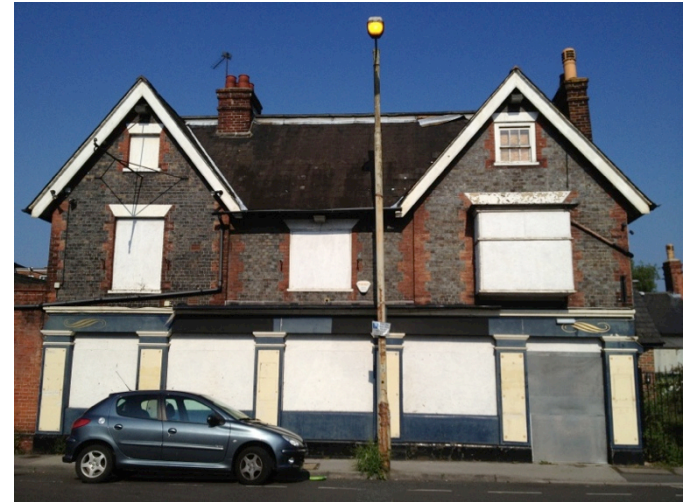
Figure 9. Existing condition of the building.
