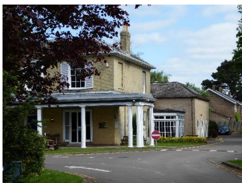
Figure B-2 View from the entrance to Denvilles House on the north side of Emsworth Road
