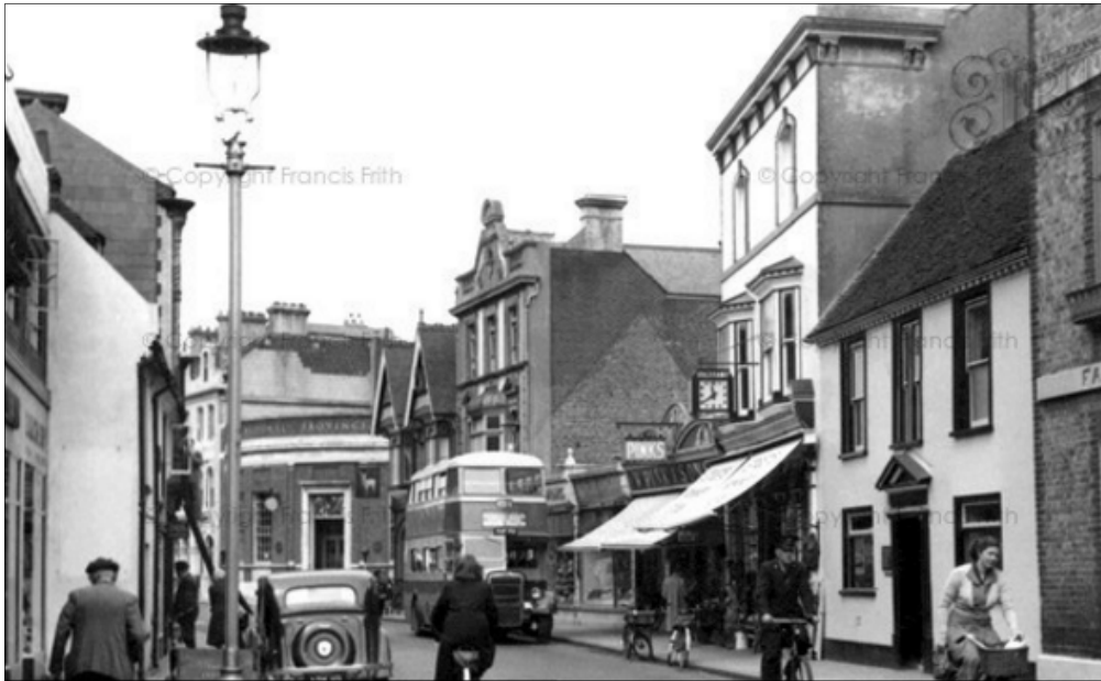
Figure 1: Westward view of N site of East St, Havant c1955 (Francis Frith Collection, negative H147007)
