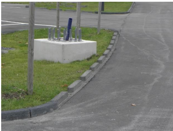
Photo 1 – Pre-Cast Foundation (other site example)
