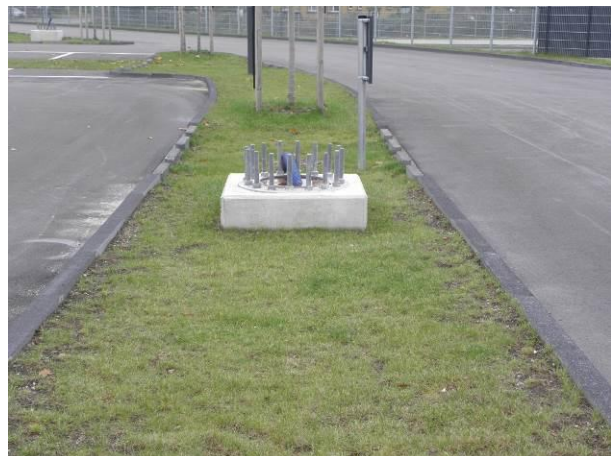
Photo 2 – Pre-Cast Foundation (other site example)
