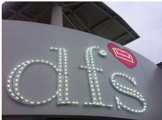
PHOTOGRAPH OF DFS LETTERS - SHOWING INTERNAL LED LIGHTS DURING CONSTRUCTION.
