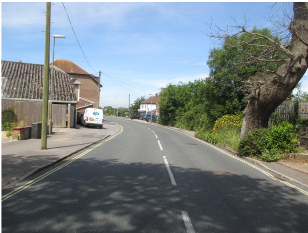
Photograph 3: Station Road Environment
