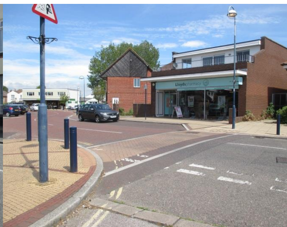
Photograph 6: West Town centre Pedestrian Environment
