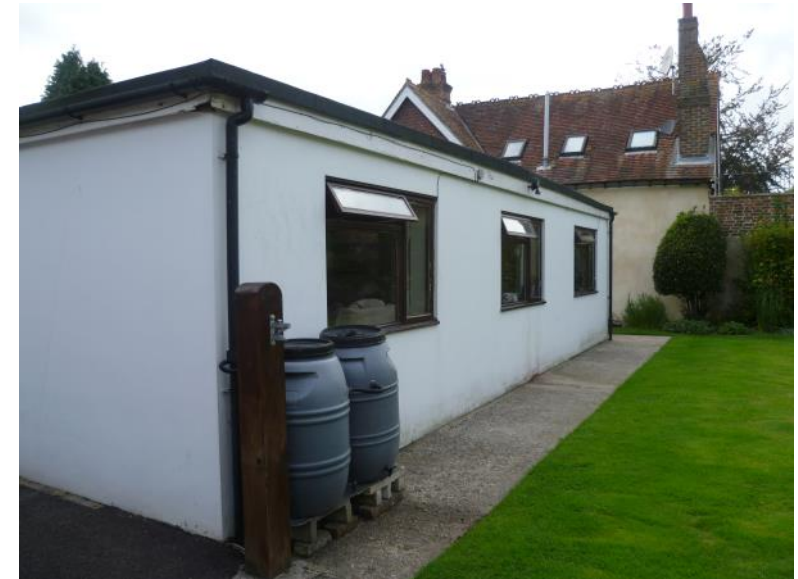
Rear Elevation & adjacent property
