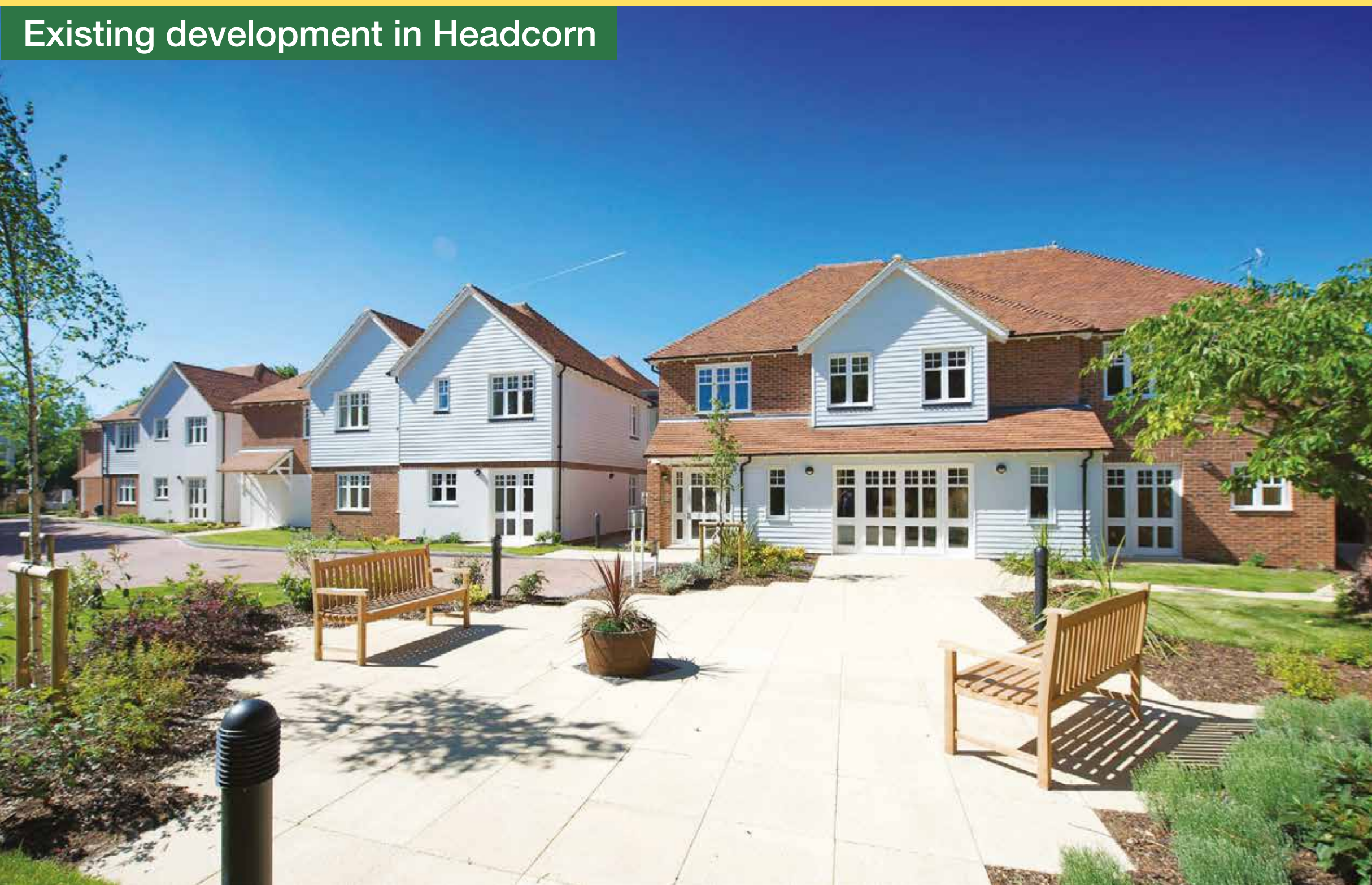
Existing development in Headcorn
