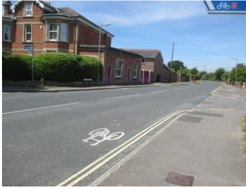
Photograph 4: Station Road on road cycle route
