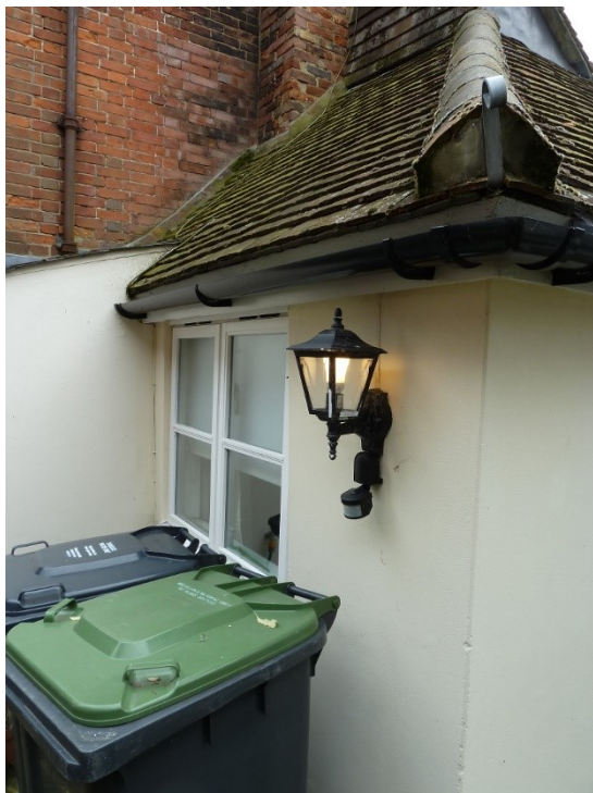
Sand-cement render to all elevations of No 22 Queen Street.
