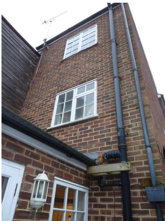
North elevation of No 18 in modern cavity construction.
