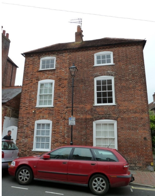
South elevation of Nos. 18 and 20 Queen Street on back edge of public highway.
