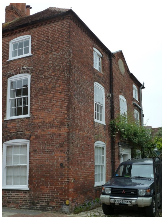
View of 20 Queen Street from the southeast with off-street parking alongside principle elevation.
