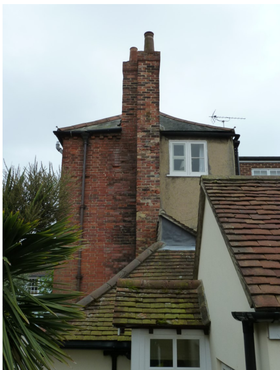
View of north elevation of 20 Queen Street with No 22 in foreground. Note attached chimney.
