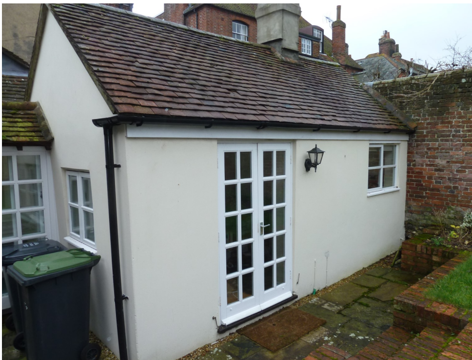
North elevation of No 22 Queen Street with modern French doors casement window. The roof is clad with C20th plain clay tiles.
