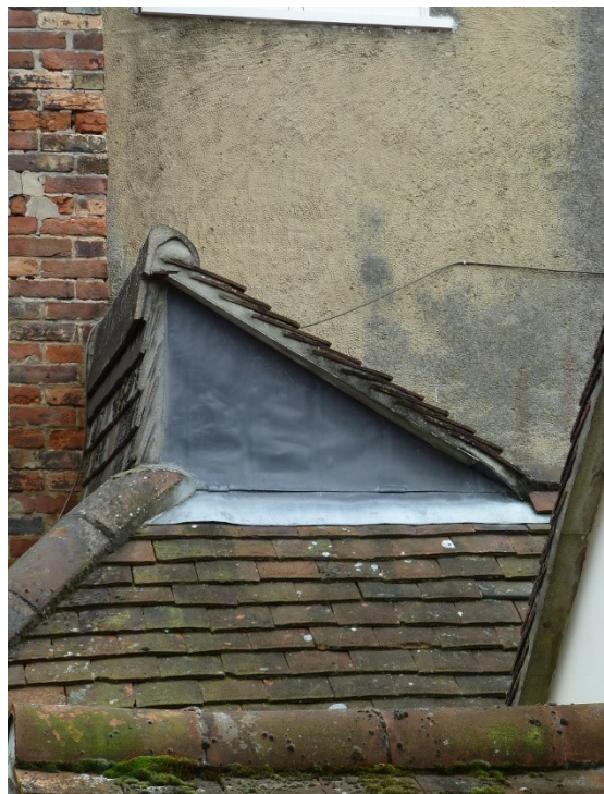
Complexity of roofs to the rear additions to Nos. 18 and 20.
