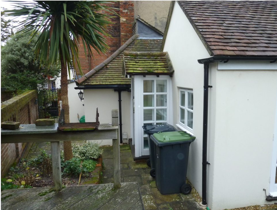
No 22 Queen Street viewed from the north. External walls are sand-cement rendered and painted. Gutters and rainwater downpipes are Upvc.
