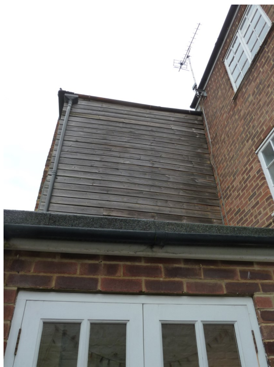
At high level lap-boarded west elevation of No 20 Queen Street.
