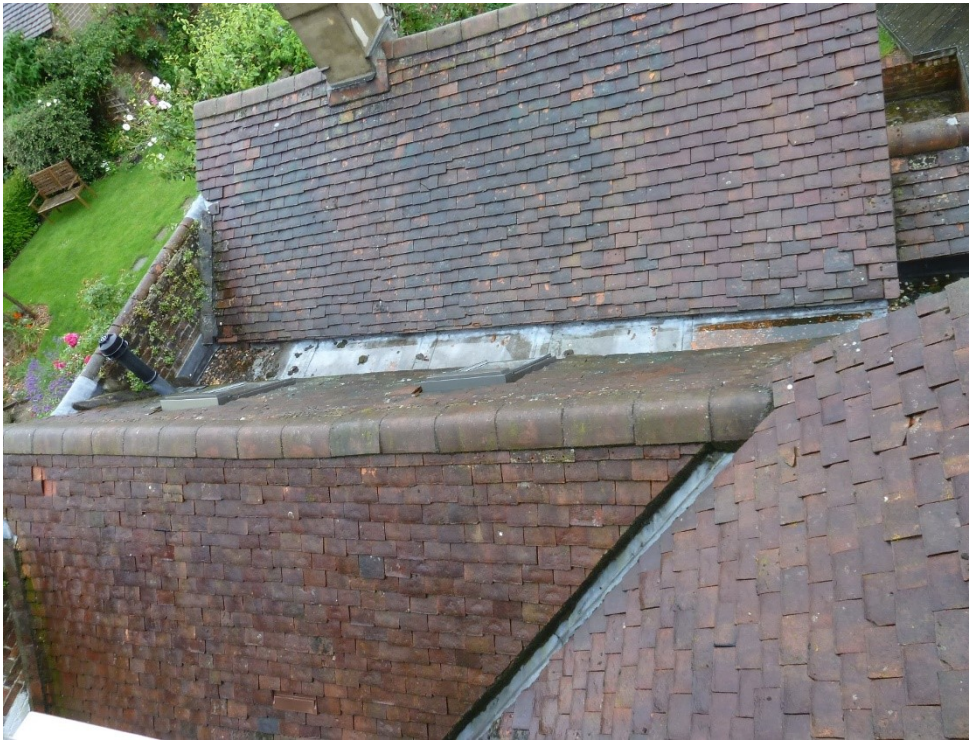
Roofs viewed from above to No 22 Queen Street clad with C20th plain clay tiles.
