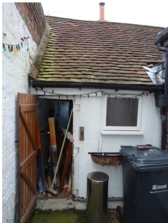
No 22 Queen Street viewed from south with bathroom window and store to No 18.
