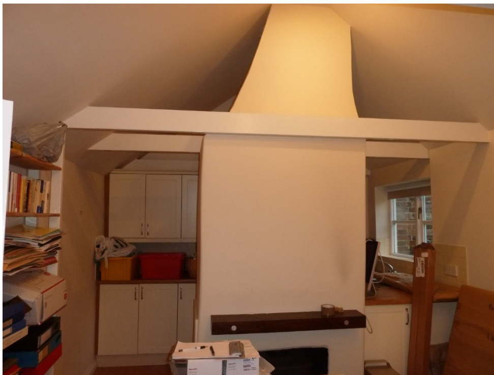
Internal view of chimney with modern plaster finishes. Modern timber collars and regular roof lines may indicate a replacement roof structure prior to tiling.
