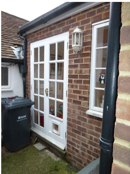
Single storey flat roof extension to No 18. abutting No 22.
