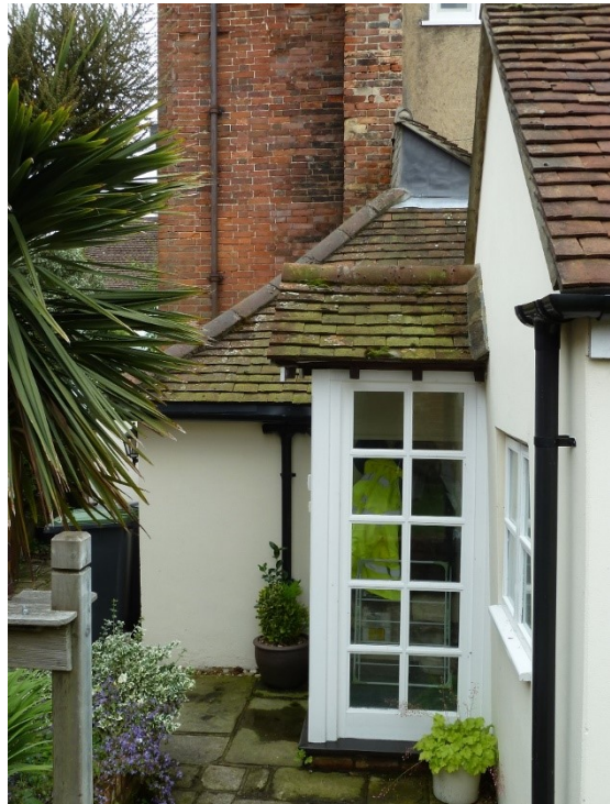
Fully glazed porch addition viewed from north.
