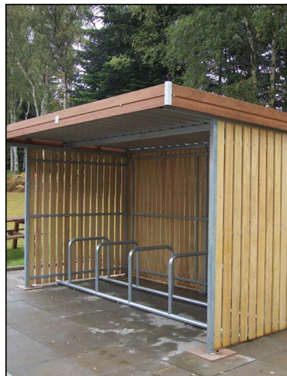
2. Cycle shelter Galvanised steel and timber slats
