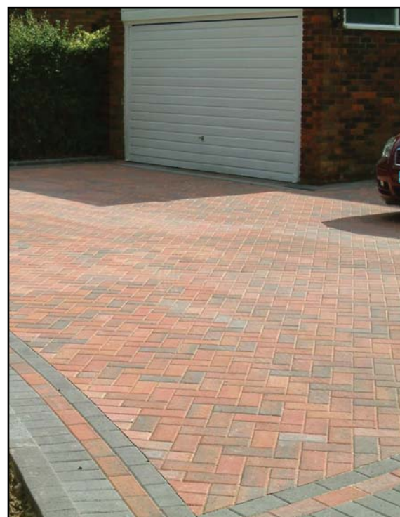
6. Concrete block paving for car park
