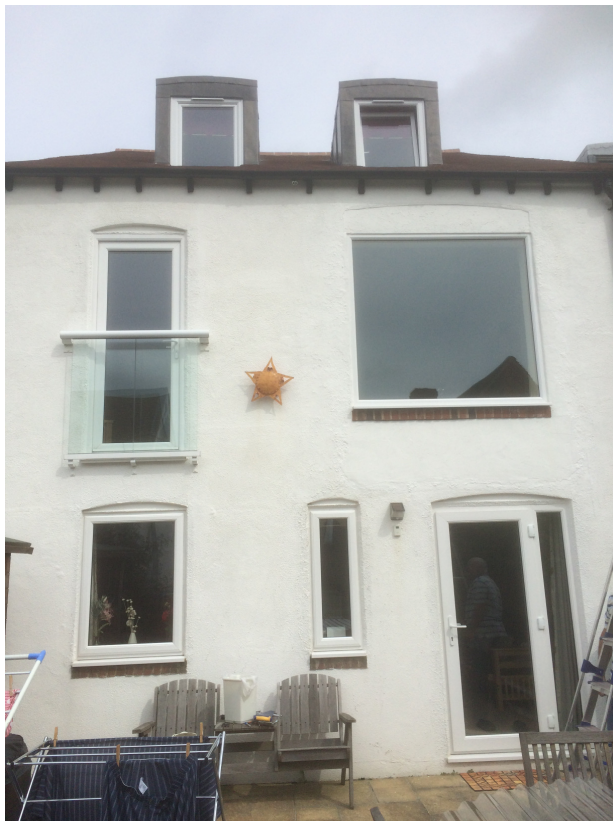
Fig 1 – Rear view of the property when viewed from the courtyard garden
