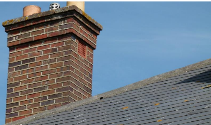
5. House roof showing generally close-fitting tiles but occasional apertures.
