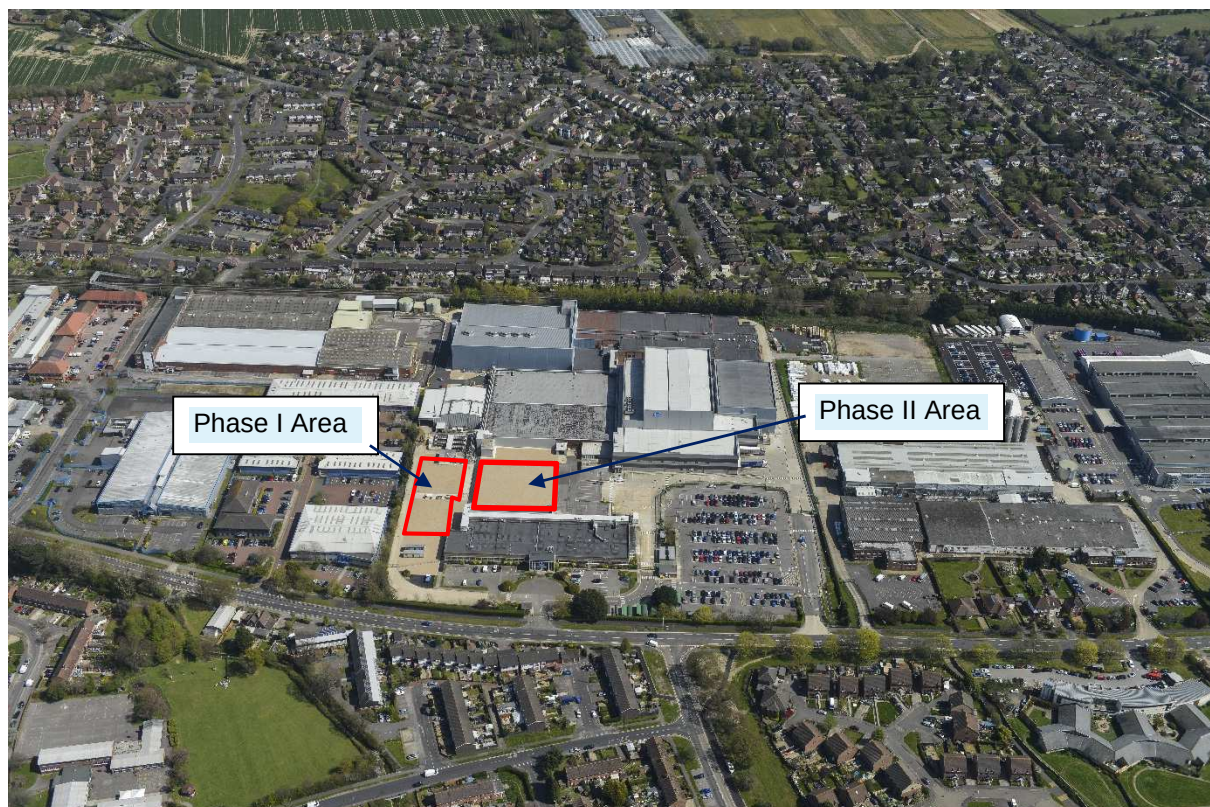
Figure 1: Pfizer Havant: Ground mounted PV Phase I & II
