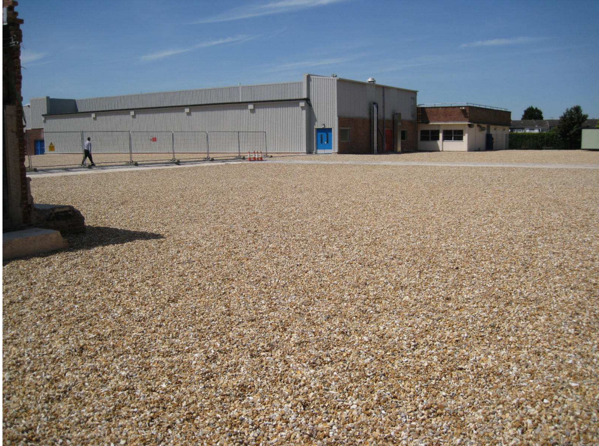
Figure 2: The development area from Substation 2/3 looking west
