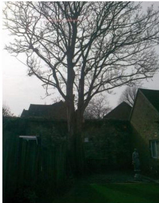
south boundary wall
