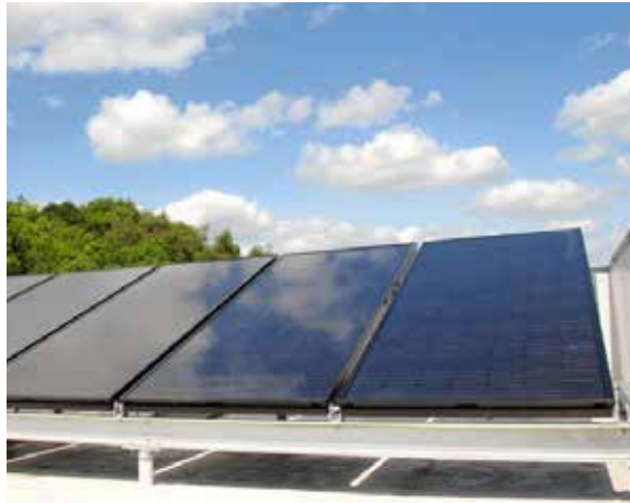
Photovoltaic array hidden behind parapet on upper roof
