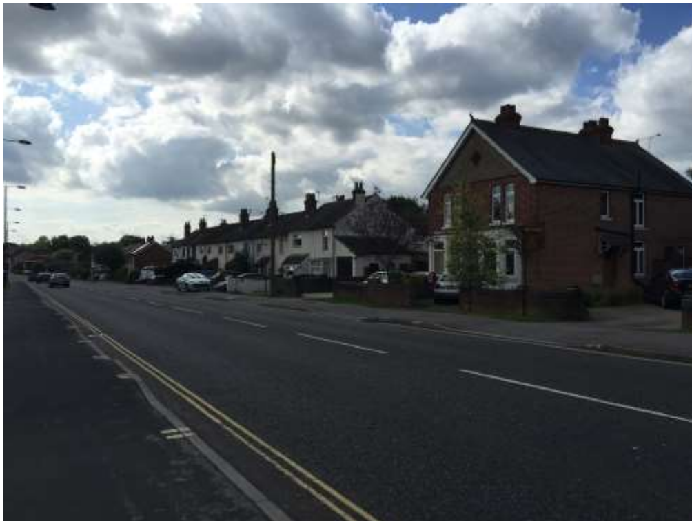
View of London Road street scene showing clear visibility and varying dwelling types and architectural styles. Within the immediate area are one and two storey properties; including detached, semi-detached and terraces all constructed of varying materials.
