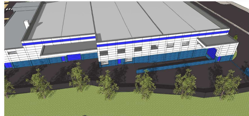
Loading Bays CGI
