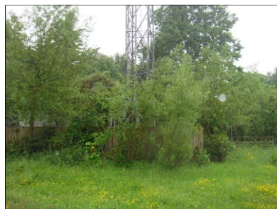
Photo 5 Mobile phone mast
