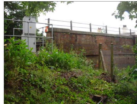
Photo 3 Railway and bridge
