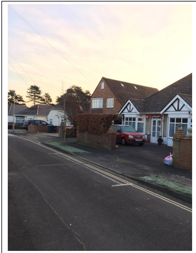
Fig. 1 - View looking to towards West Elevation
