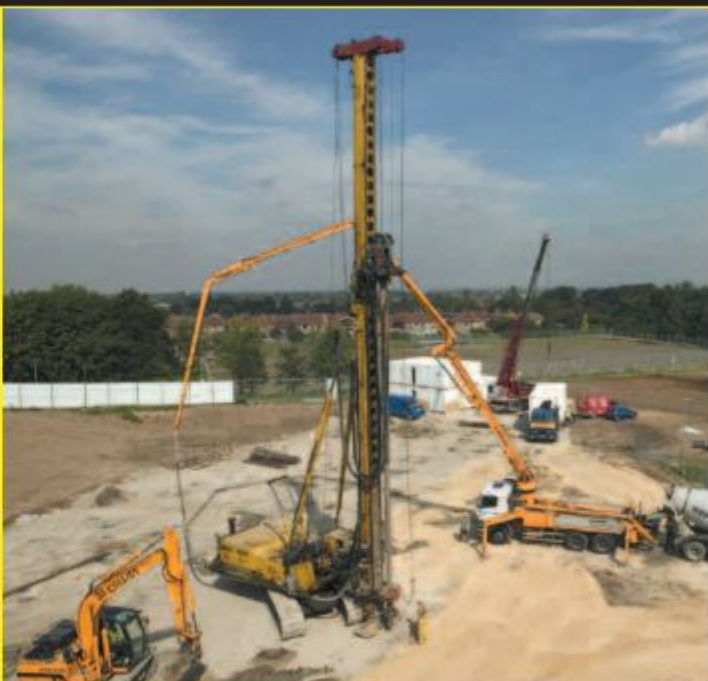
CHD piles being formed at a large unrestricted construction site
