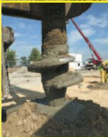
Completion of the concrete procedure in readiness for the steel reinforcement. N.B. Minimal soil arisings
