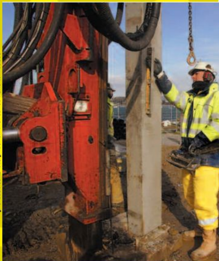
RB 5000 series rig incorporating the RB "Quiet" Hammer, installing 200mm square pre-cast concrete piles for the foundations to houses
