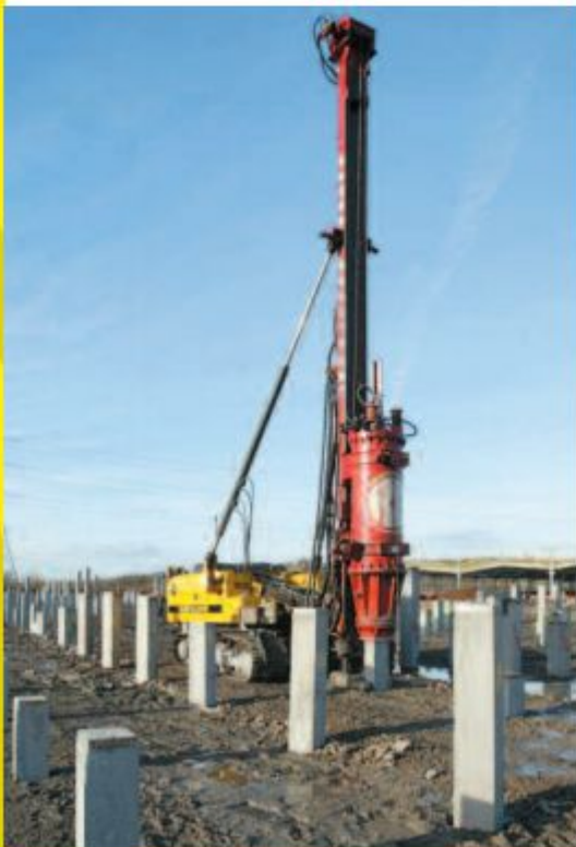
RB 5000 series rig can install 250, 275 and 300mm square pre-cast concrete piles
