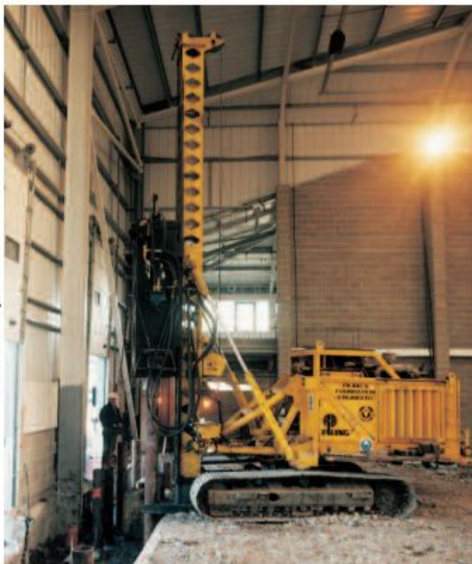
RB 5000 series driven piling rig installing steel tubular piles, adjacent to the external wall, within a warehouse
