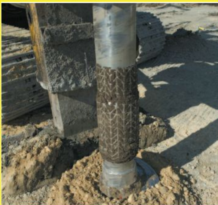
Drilling procedure initiated
