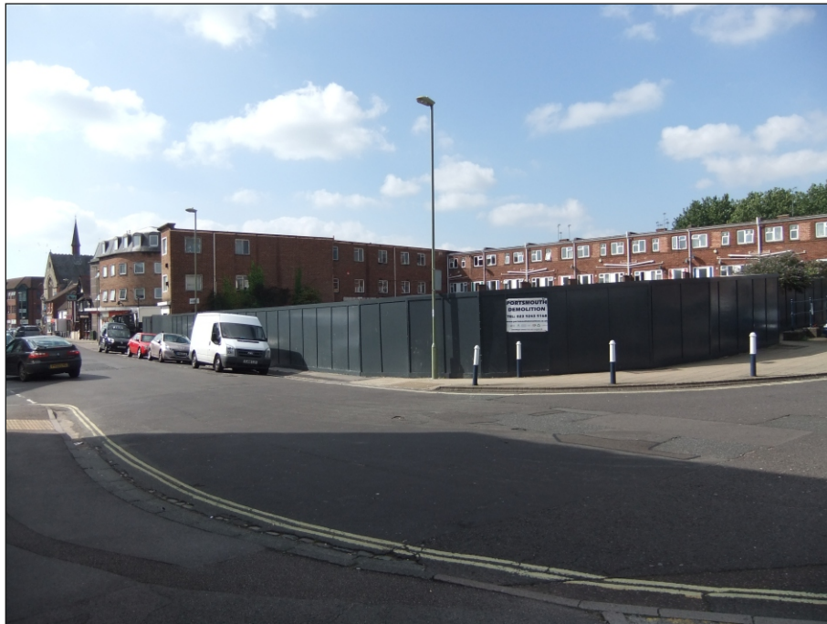
Plate 3: View from north-east across Site
