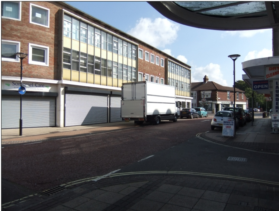
Plate 1: Southern facade of current building on Site
