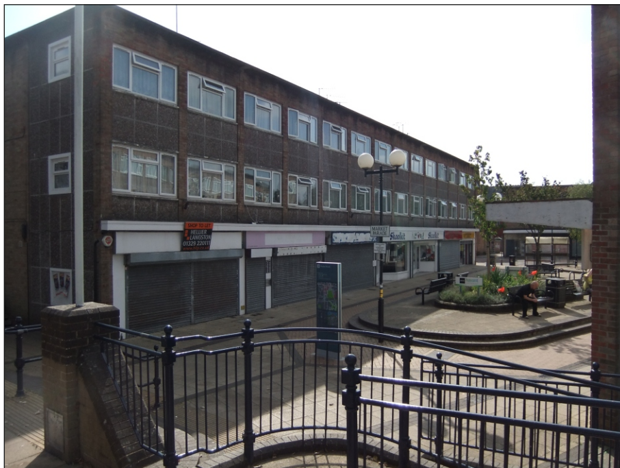
Plate 4: Western facade of current buildings on Site and pedestrian plaza
