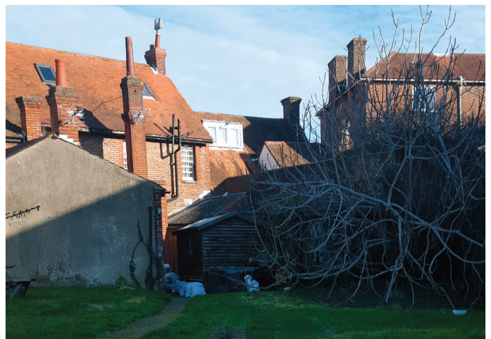
Rear view of 1 High Street
