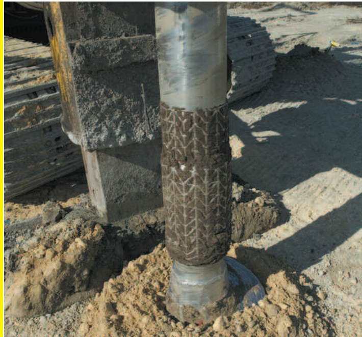
Drilling procedure initiated
