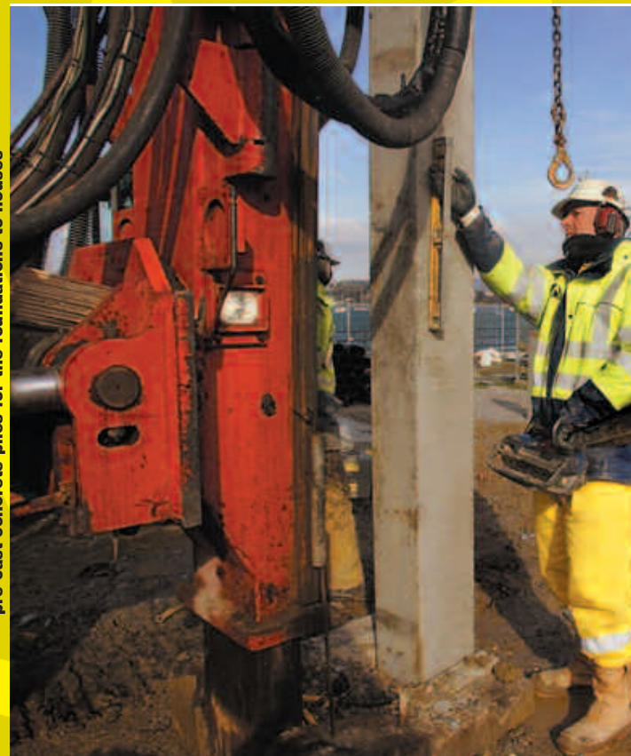
RB 5000 series rig incorporating the RB "Quiet" Hammer, installing 200mm square pre-cast concrete piles for the foundations to houses
