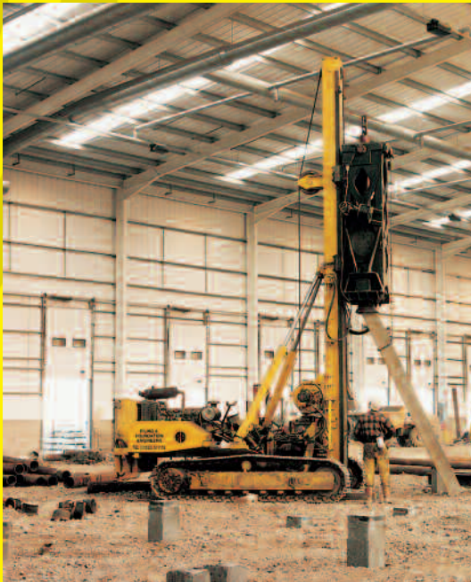
RB 5000 series low-headroom rig installing 250mm square pre-cast concrete piles inside an existing warehouse to provide additional support for a new floor slab
