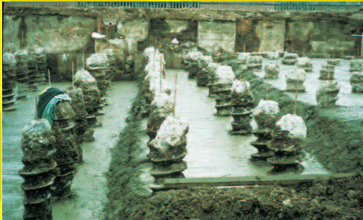
Completed CHD piles awaiting basement floor construction
