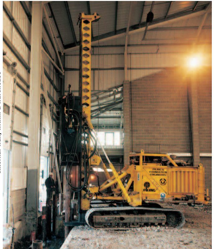
RB 5000 series driven piling rig installing steel tubular piles, adjacent to the external wall, within a warehouse
