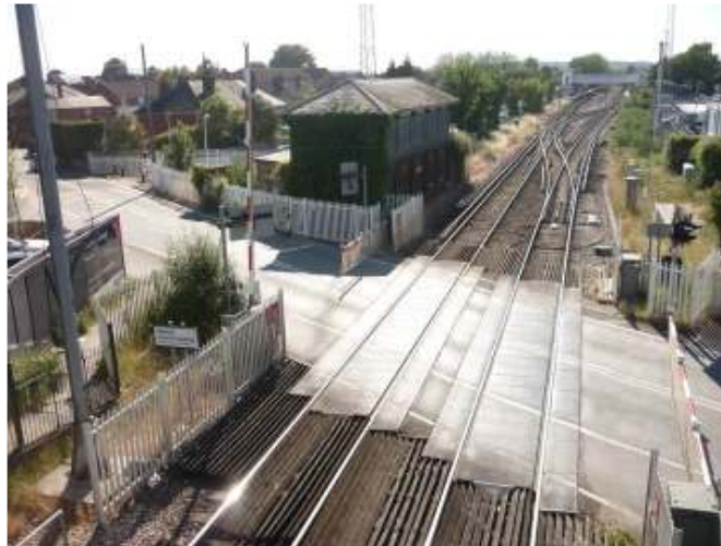
Fig 11: Grade 2 listed Signal Box to the South west of site
