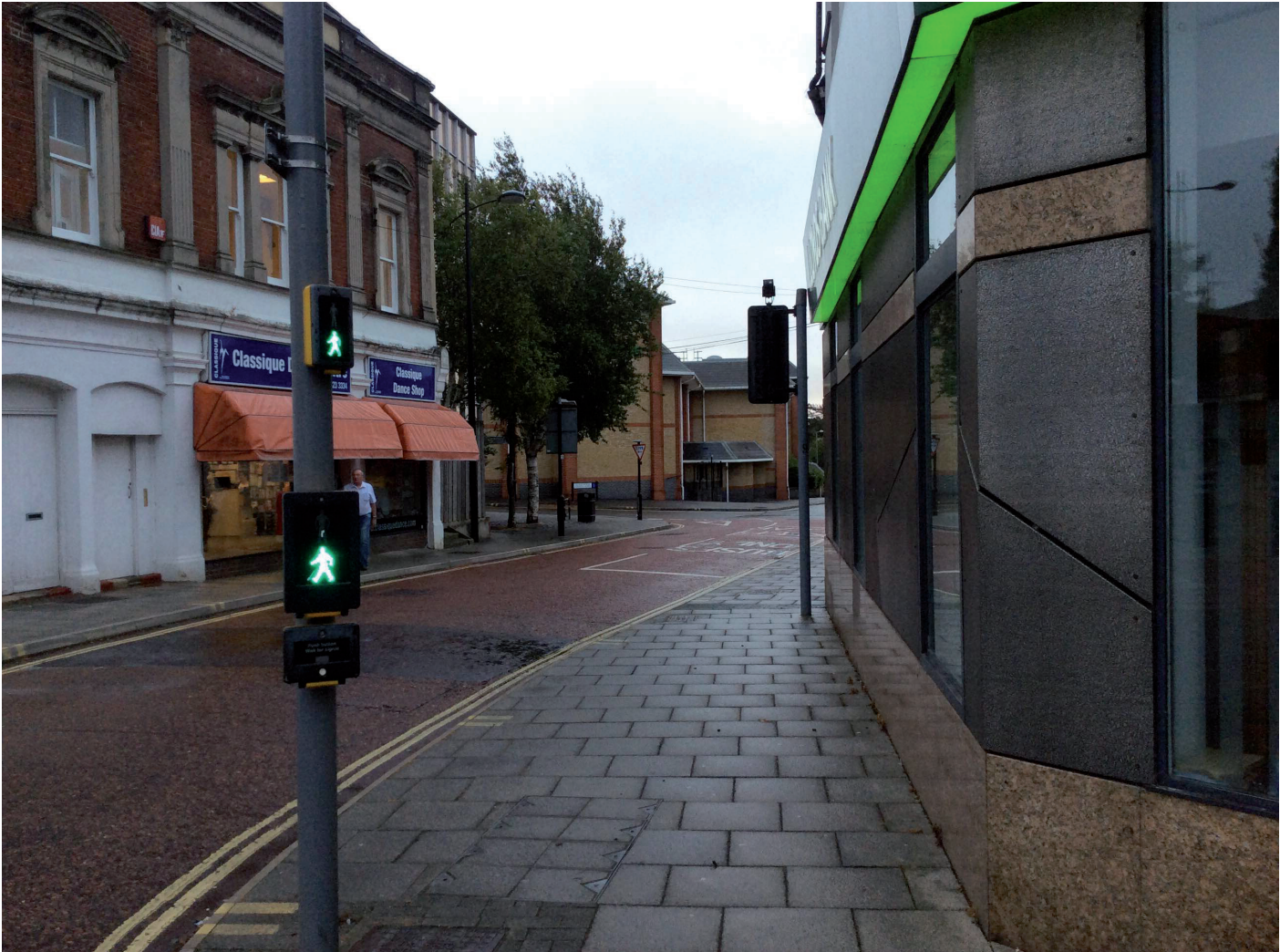
Existing view from high street approaching from the north
