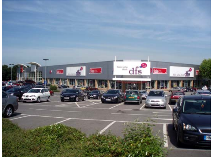
View of DFS Unit
