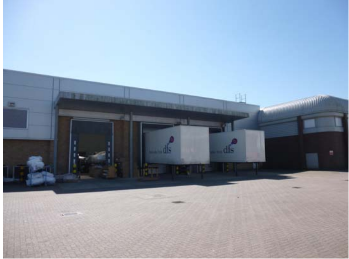
Existing rear service area to DFS
