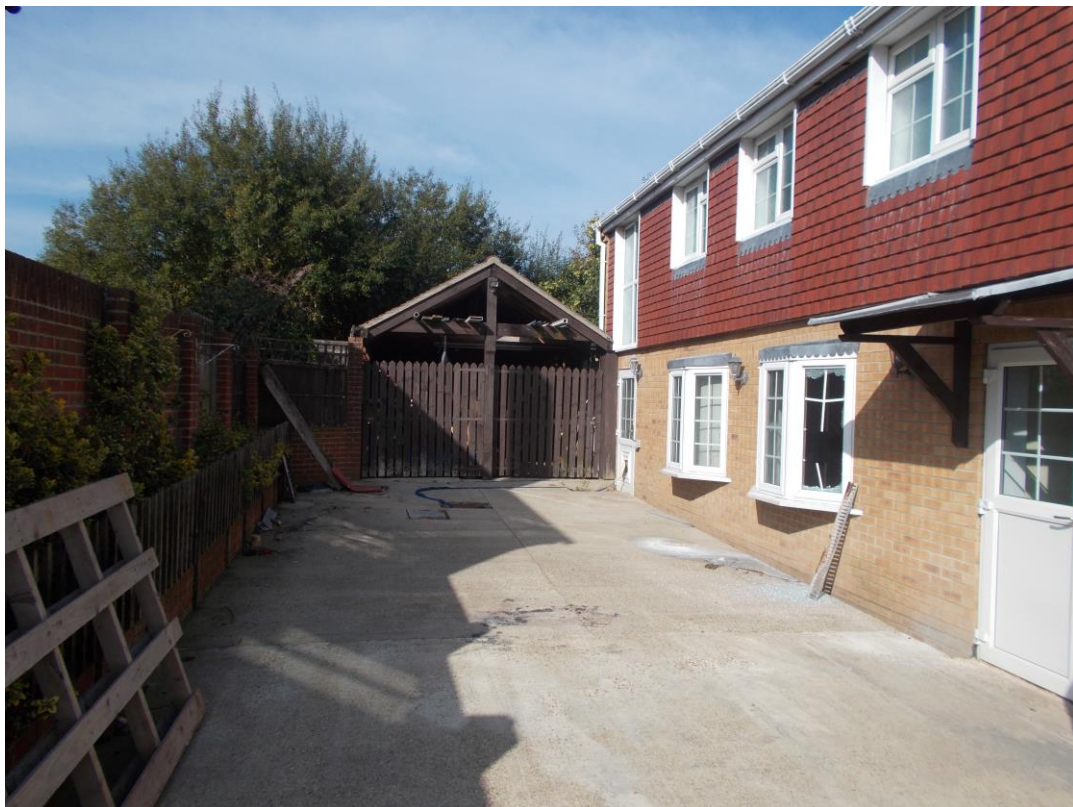
Figure 3. The hardstanding and garage.
