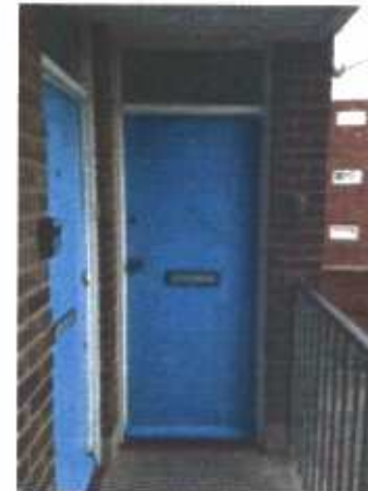
House 5 Door - South Elevation
