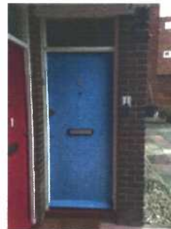
House 1 Door - South Elevation
