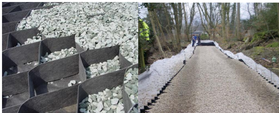
Figure 4. Photographs illustrating cellular confinement system used to form an above-ground no-dig driveway
