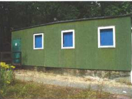
Port Cabins South-East Elevation
