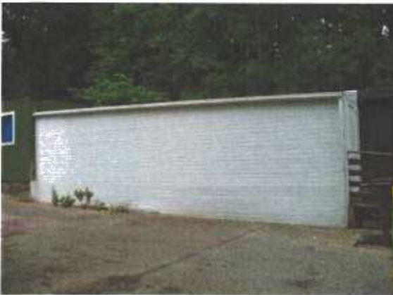
Port Cabins South-East Elevation
