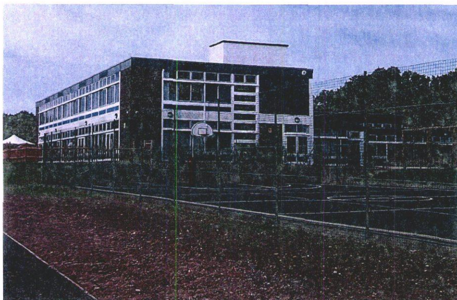
Plate 4 – School buildings and hard standing play surfaces on site
