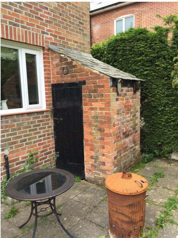
Figure 9: Existing coal shed to be demolished and rebuilt as existing
