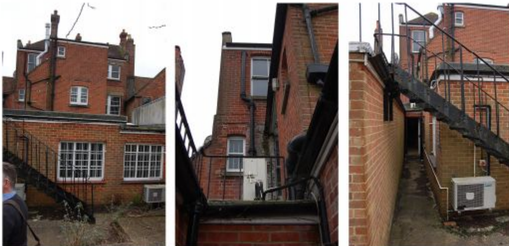
Images of the rear of the building
