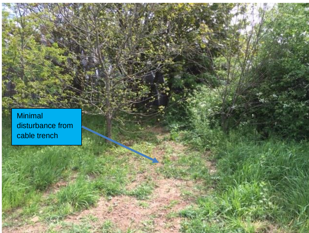
Photo 7 – Cable trench route through grassland and hedge
