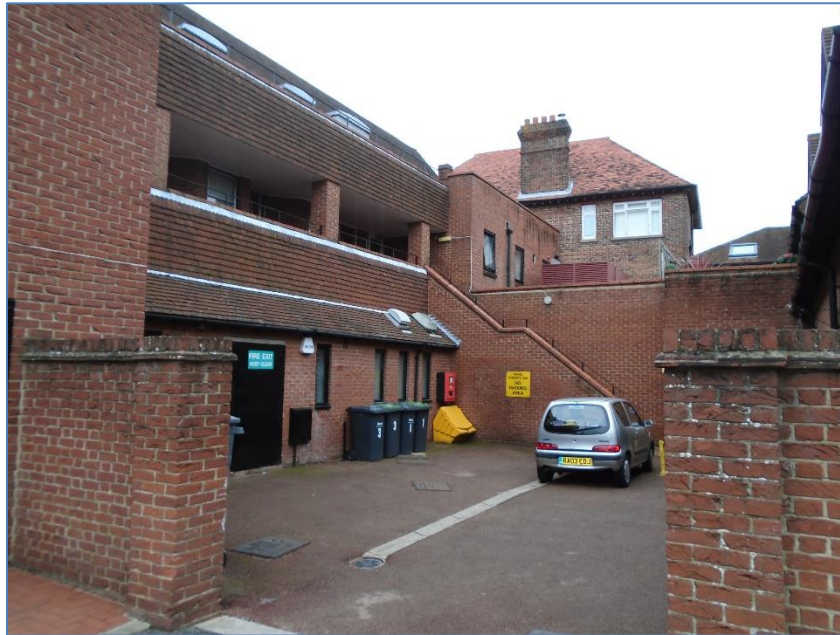
Bin store location to the rear of the unit
