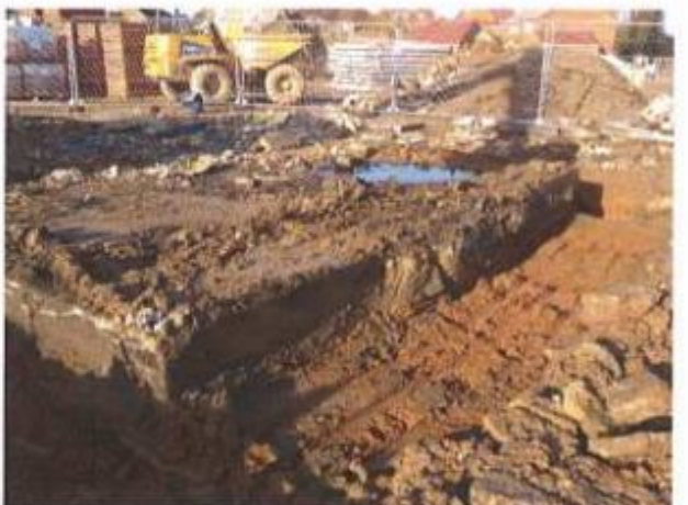
Photograph showing tank base prior to removal
