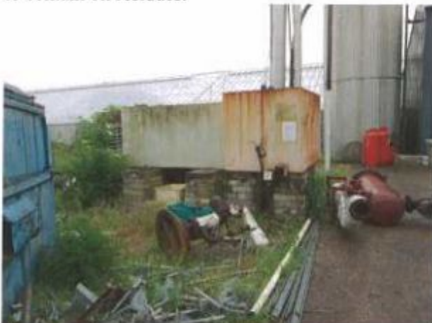
Photograph showing some of the disused oil tanks located to the east of the main boiler house prior to demolition.
