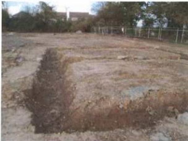
Photograph showing area of former above ground heating oil tank
