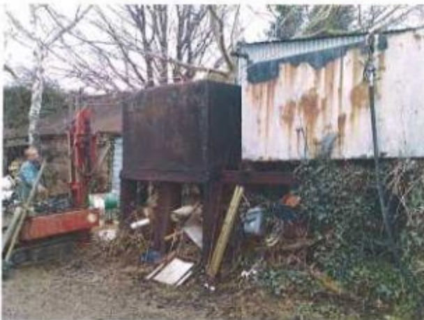
Photograph showing the tanks -note the adjacent ground investigation borehole that encountered low level hydrocarbon contamination
