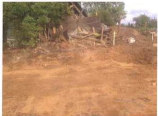
Photograph showing the former location of tank base excavation following removal
