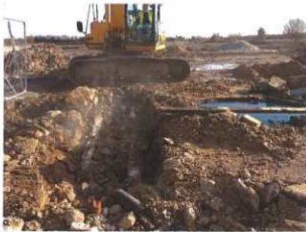
Photograph showing the removal of the base and short section of duct
