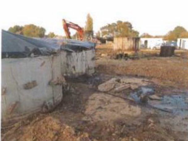
Photographs showing oil tank base during the early stages of demolition
