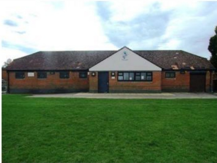
Photograph 9: View of the front northern elevation of the Pavilion.
