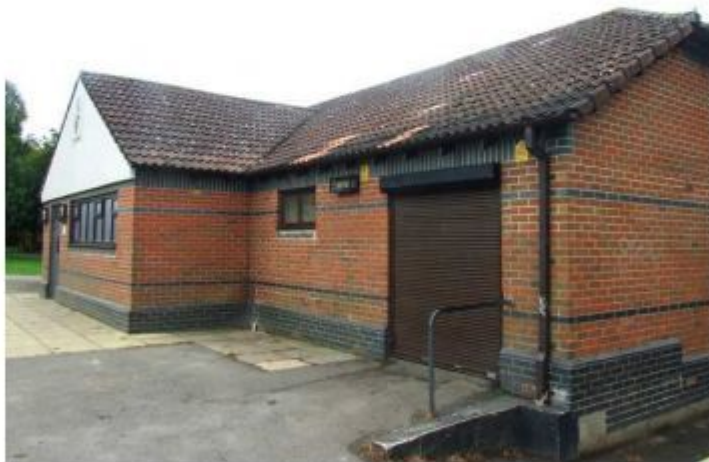
Photograph 11: View of the cross gable of the pavilion.
