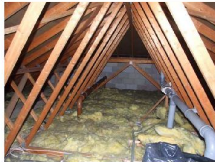
Photograph 12. The interior roof space.
