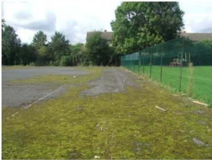
Photograph 5: The existing hard standing tennis courts.
