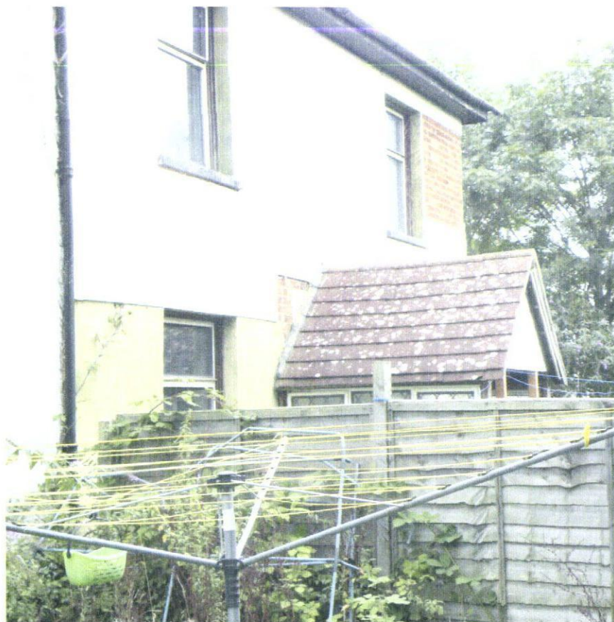
Photo 3 South Elevation 71 Third Avenue
