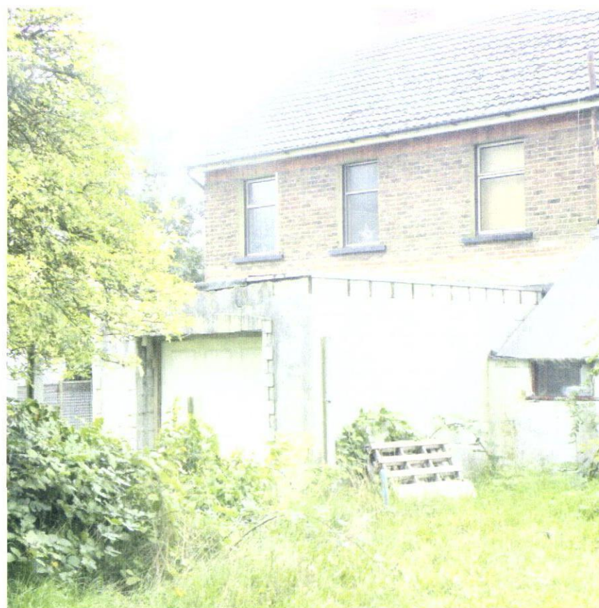
Photo 4 North Elevation of 71 Third Avenue from 73
