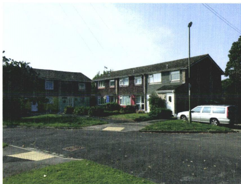
Photo 6 View of Third Ave looking South-west
