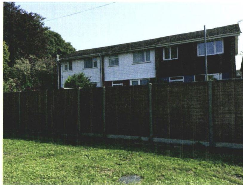
Photo 8 View of 65 to 69 Third Ave from rear
