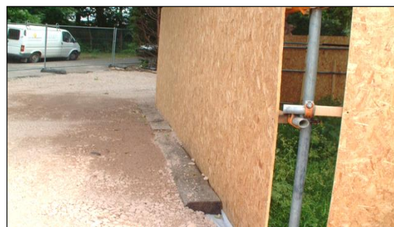
Photo 27: Although this is only a temporary surface, railway sleepers pinned into the ground can be used to retain the edges of new surfacing.
