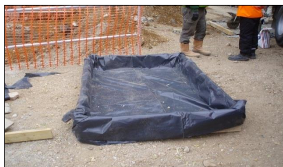
Photo 47: Soil bunding or a supporting framework covered in heavy-duty plastic sheeting is essential where there is a risk of spillages contaminating RPAs.
