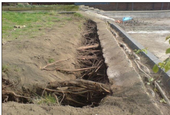
Photo 17: Air spades are particularly useful where roots are very dense.
