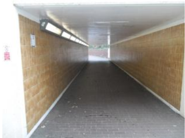
Photo 4.2: Maurepas Way underpass
