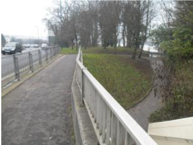
Photo 4.1: Access ramp to Maurepas Way underpass
