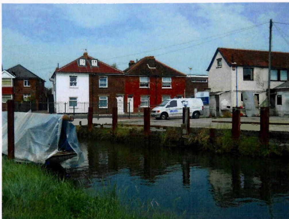
Queen Street Coastal Defence Perimeter Wall #7 location
