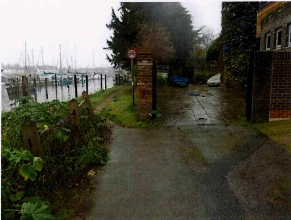
Queen Street Coastal Defence Perimeter wall #7/Ramp #8 location
