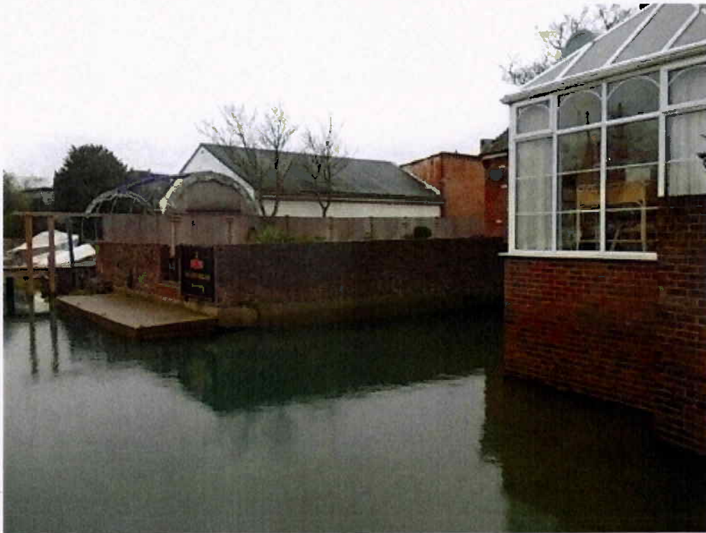
Queen Street Coastal Defence Perimeter Wall #6
