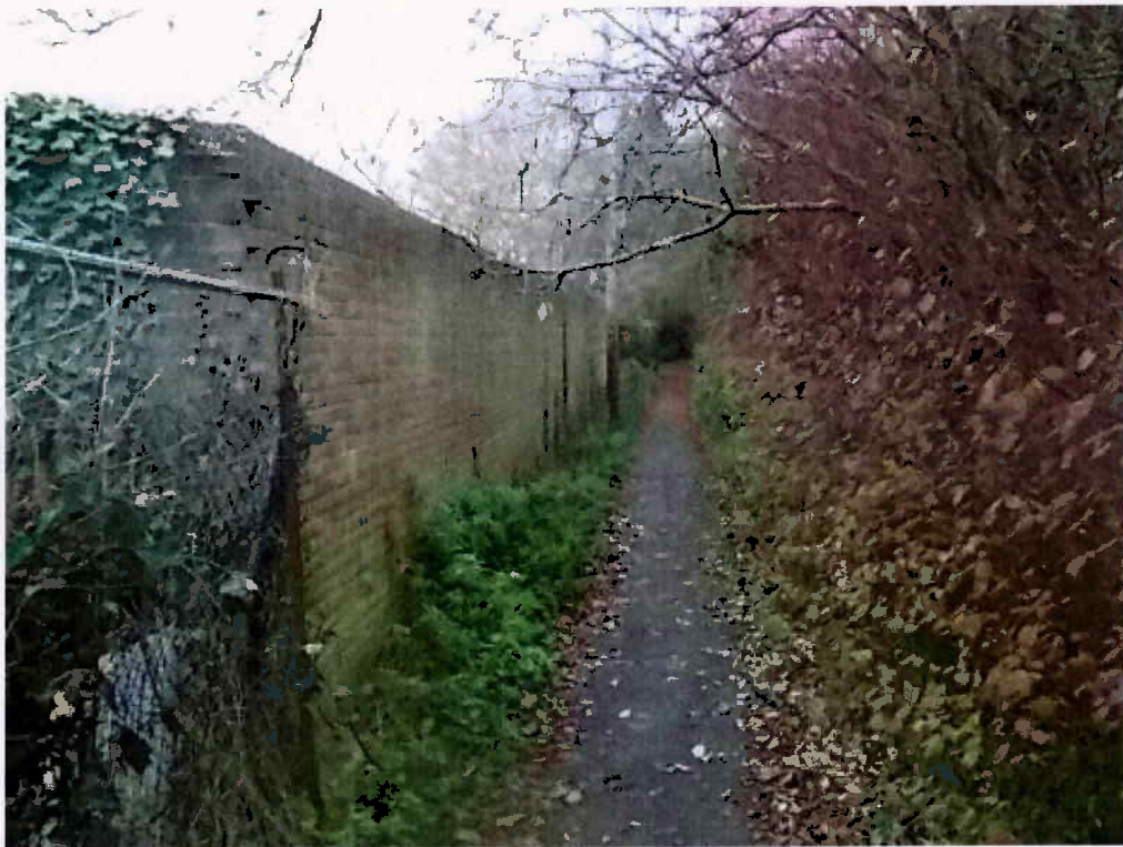
Queen Street Coastal Defence Perimeter Wall #2
