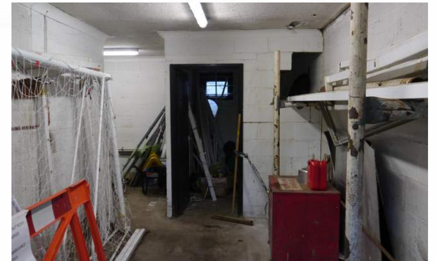
Fig 10. Internal Photograph - Storage Room
