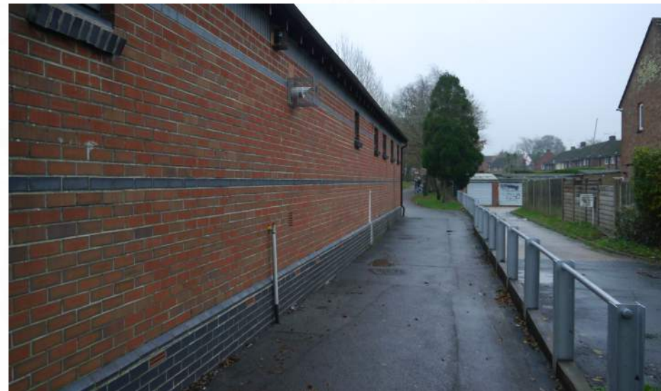
Fig 3. Photograph showing rear of existing pavilion
