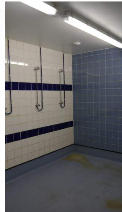
Fig 9. Internal Photograph - Existing Shower Room
