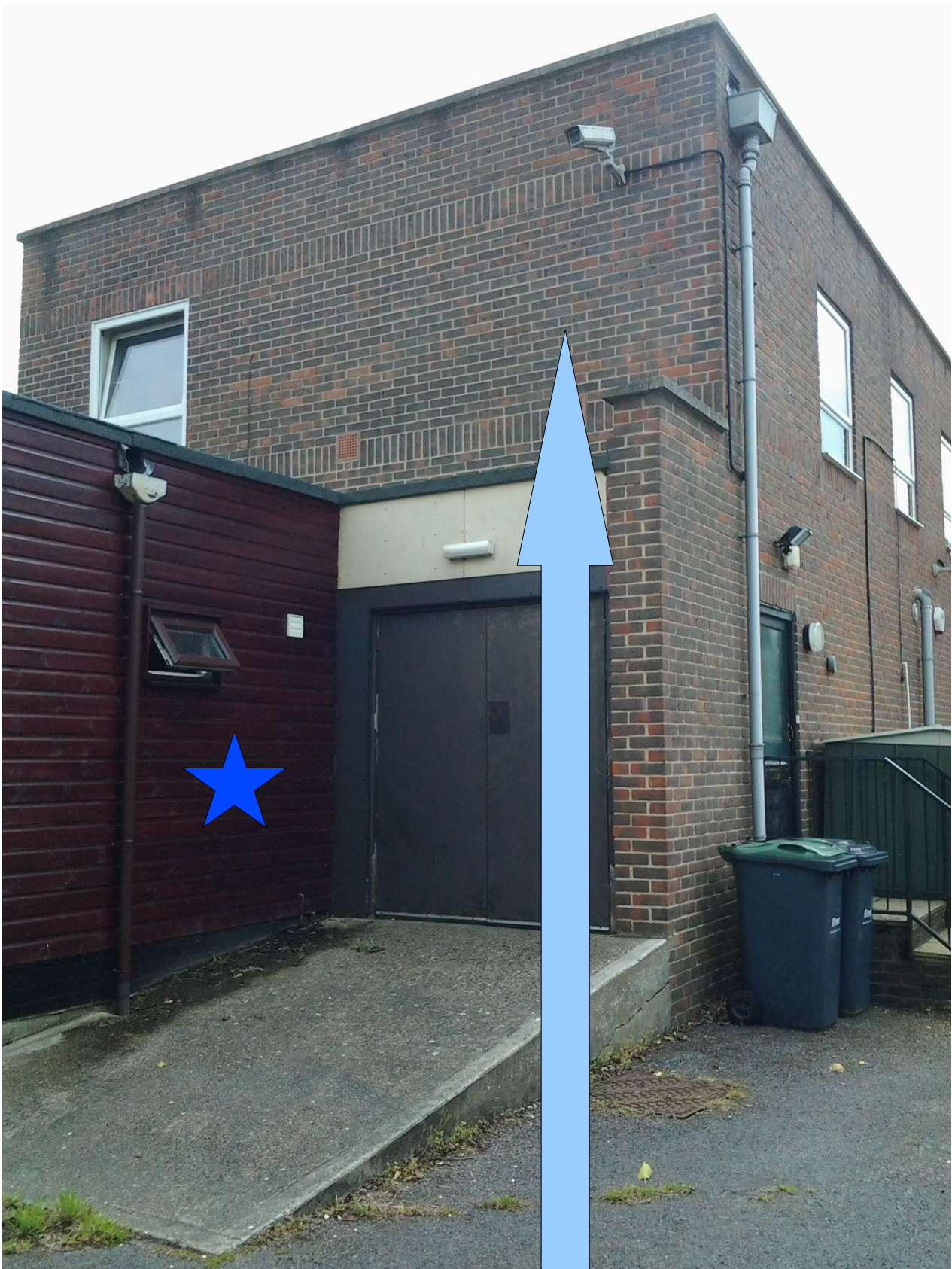
The stewards flat. The only two storey element of the existing building
