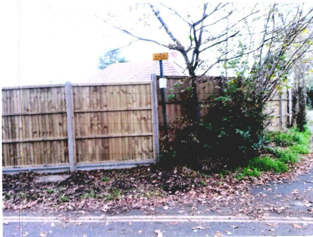
(5) 25 Bound Lane last 2 panels of new fence, driveway to no. 27
