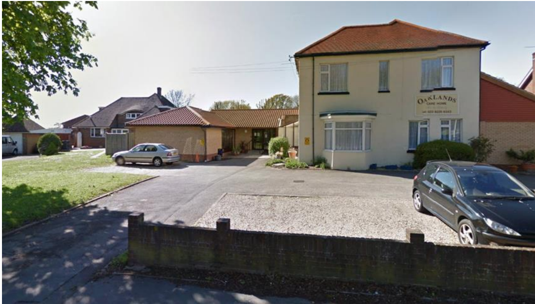
Fig. 5: View from Stakes Hill Road. (Google Streetview)
